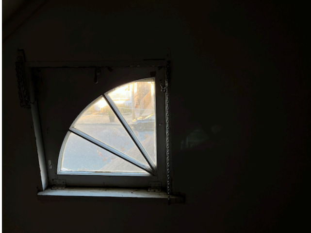
window from attic interior
