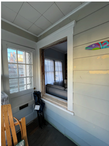
historic siding on south wall of sunroom (note previous porch floor) and door into house
