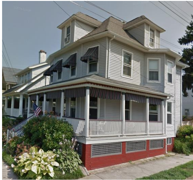
Front / Side (South-West)
