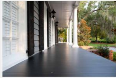
An Aeratis Traditions installation. Click here for the Aeratis photo gallery.
