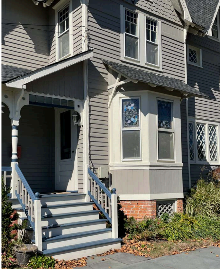
Above: 42 Abbott Avenue – Shingles, clapboard, vertical flush boards on a Queen Anne style house. Right: 63 Webb Avenue – Patterned shingles & clapboard on a Queen Anne style house. JWF Photo October 2021
