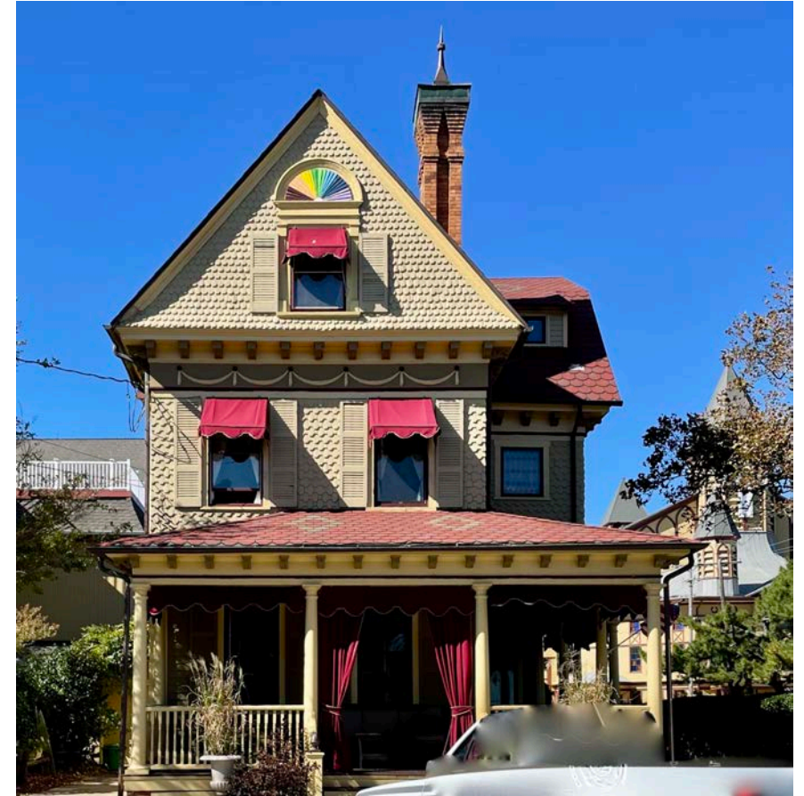
Shed dormer on "ell" projection to side
