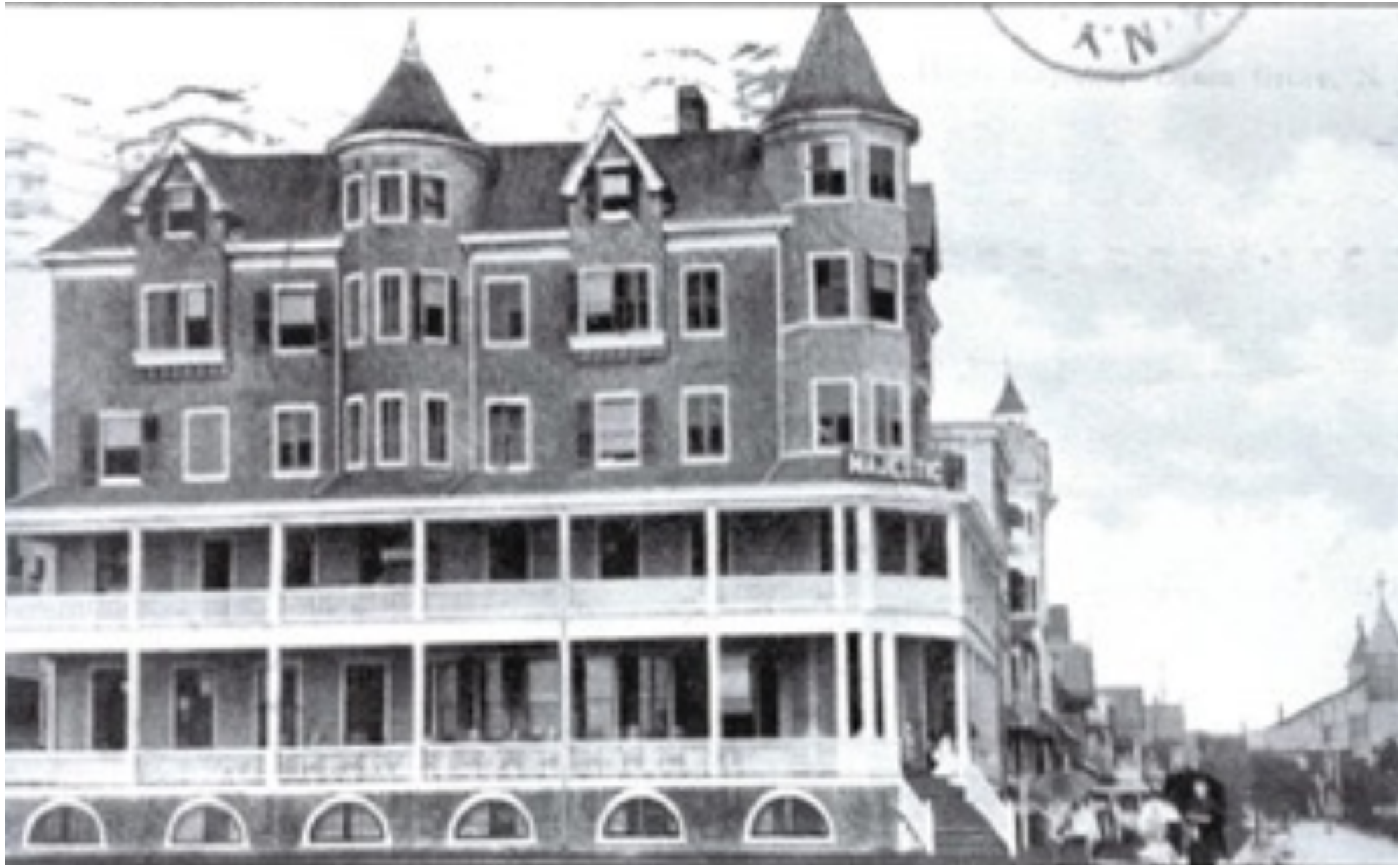
Majestic Hotel, 2 Ocean Pathway; Ocean Avenue elevation in an undated photo from Images of America: Ocean Grove
