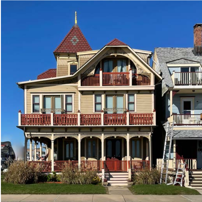
Shed dormers on front gable
