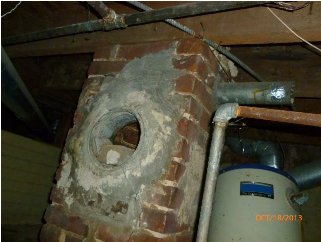
Photo 3 – Basement: Flue packing material ( note : identified to be non-ACM).
