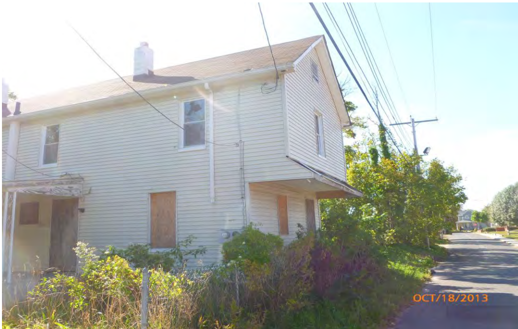
Photo 2 - General view of the subject building (side).
