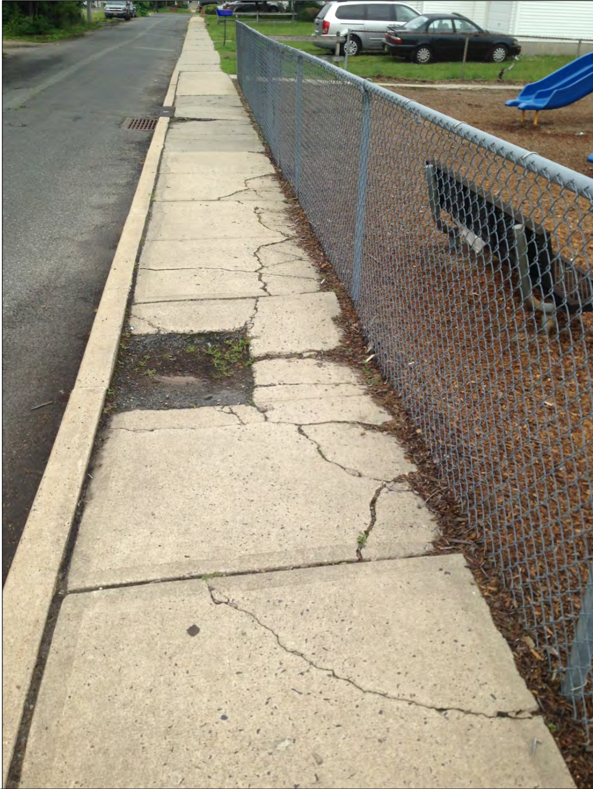
Sidewalk on north side of Division Street
