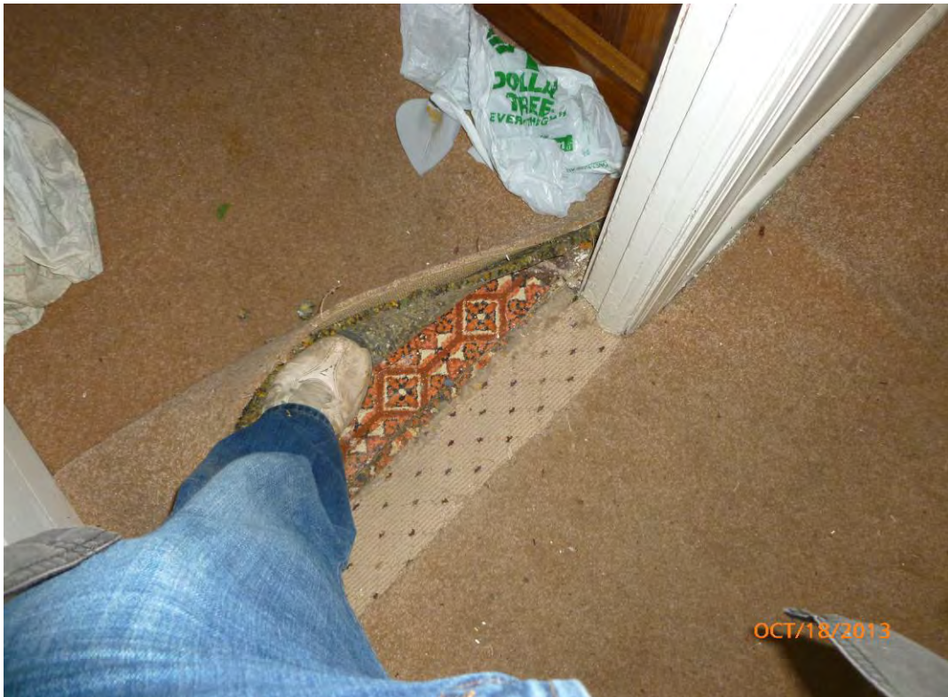
Photo 4 – 2 ND Floor Bedroom: Red linoleum ( note : identified to be non-ACM).
