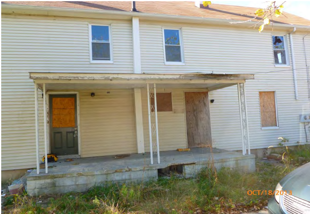
Photo 1 - General view of the subject building (front).
