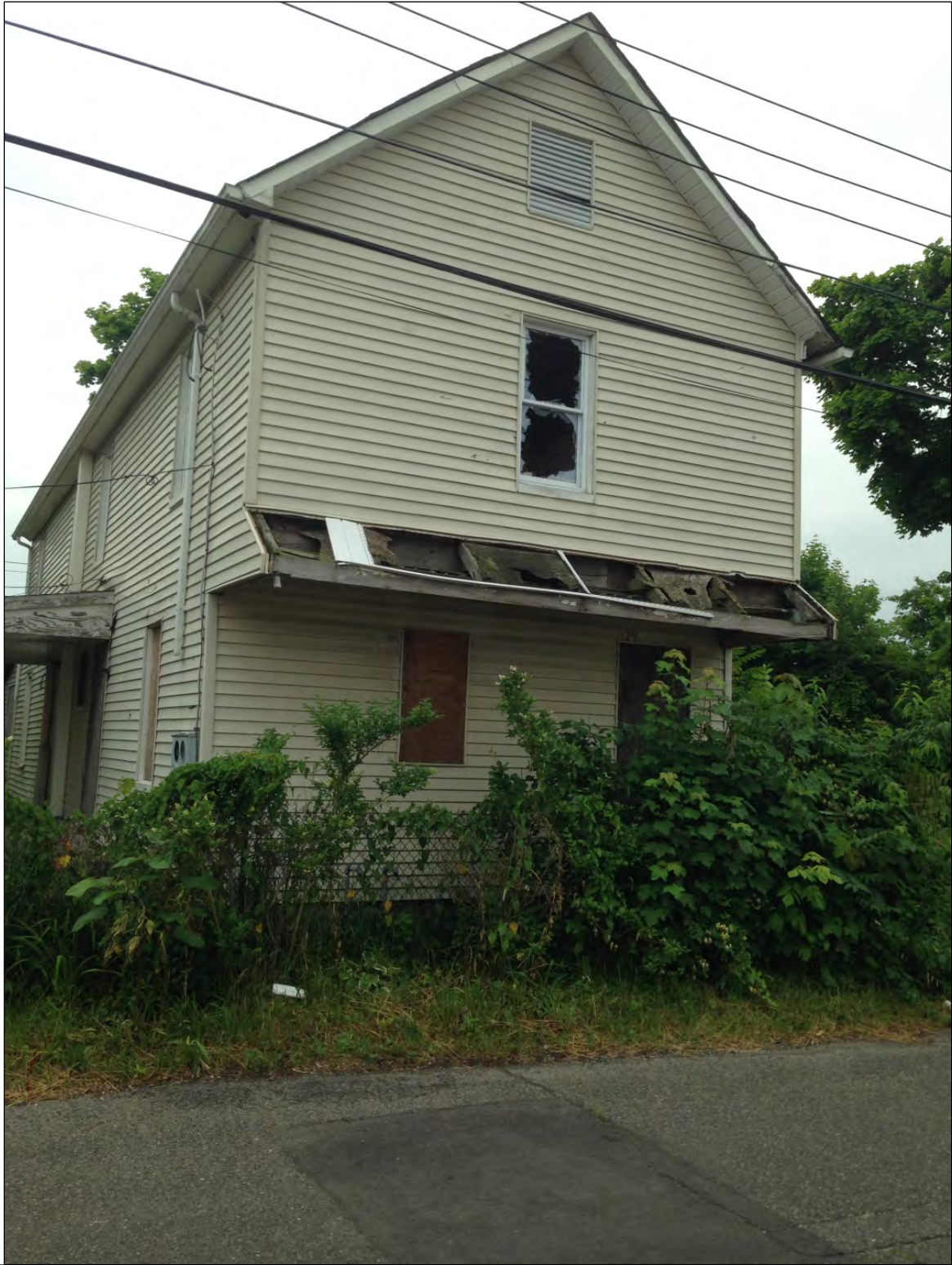
Lot 30.01: Vacant house, front angled view.
