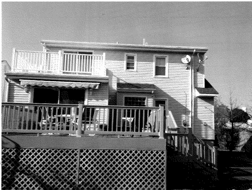
REAR VIEW 21 ALBANY ROAD NEPTUNE, NJ AUGUST 5, 2014
