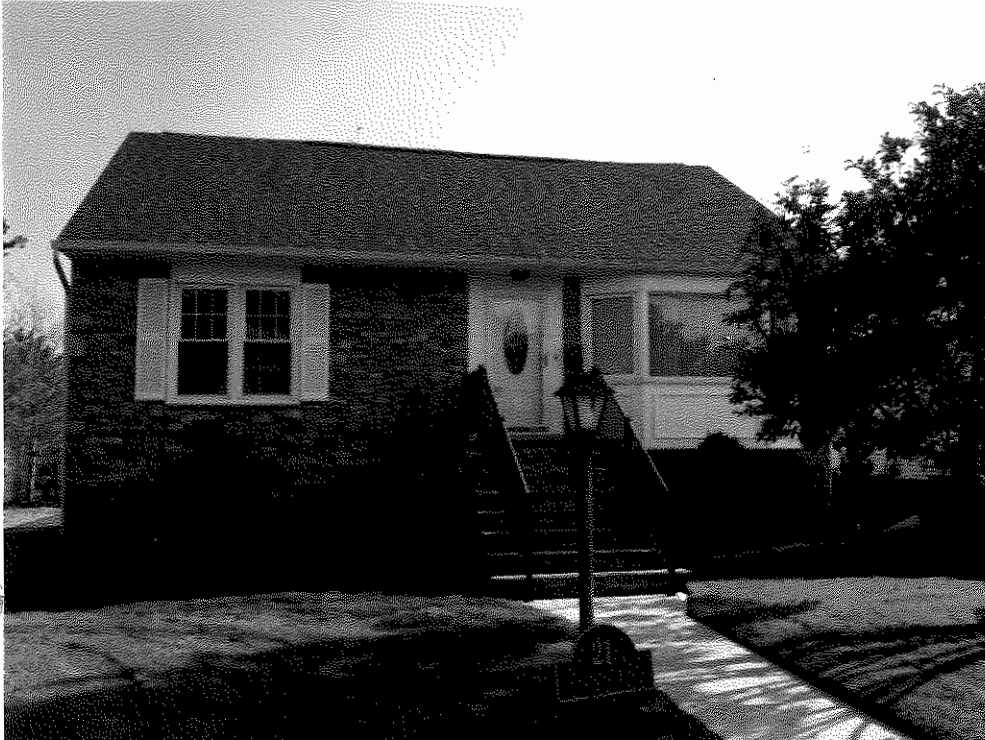
FRONT VIEW 21 ALBANY ROAD NEPTUNE, NJ AUGUST 5, 2014
