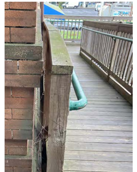
View from Upper Ramp Landing
