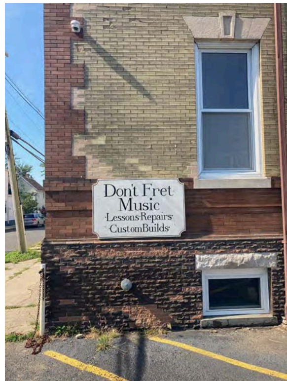
North Facing NE Corner Elevation (am sun)
