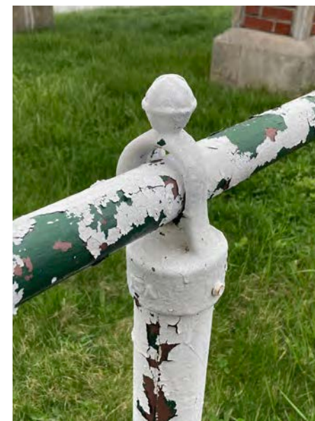
Post Head Cap & Rail Eye Detail 2
