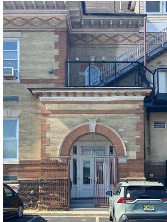
North Entrance (Main Avenue)
