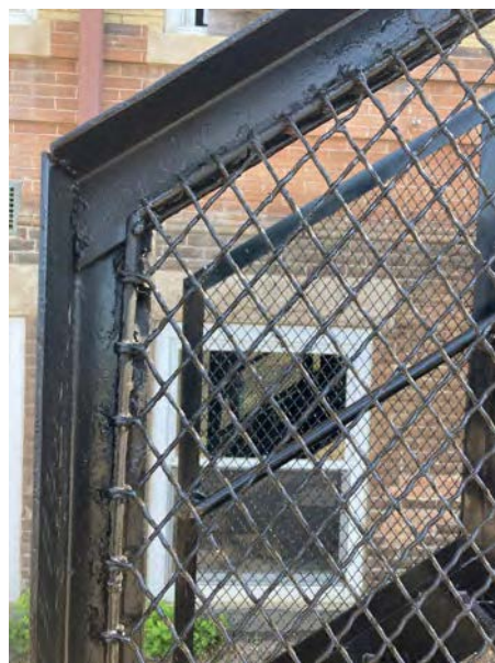
Welded Mesh Detail
