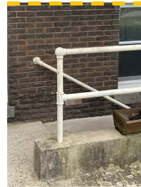
2. Rail to Below (Northwest)
