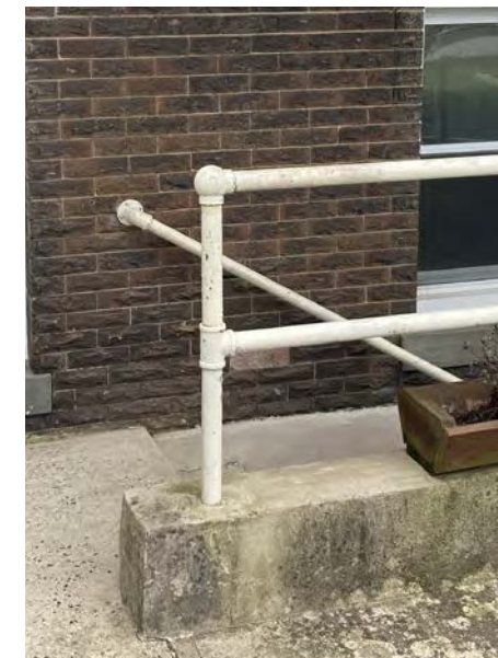
2. Rail to Below Detail (Northwest)
