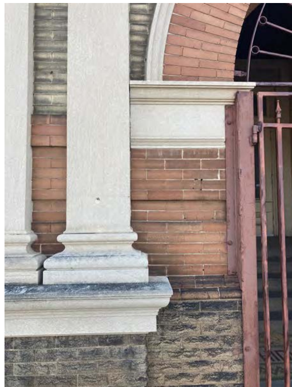
Detail at West Entrance Gate (am sun)
