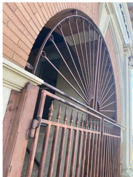
West Entrance Gate
