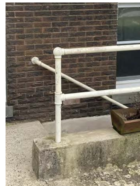
2. Rail to Below (Northwest)
