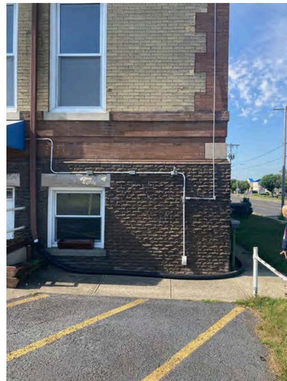
North Facing NW Corner Elevation (am sun)
