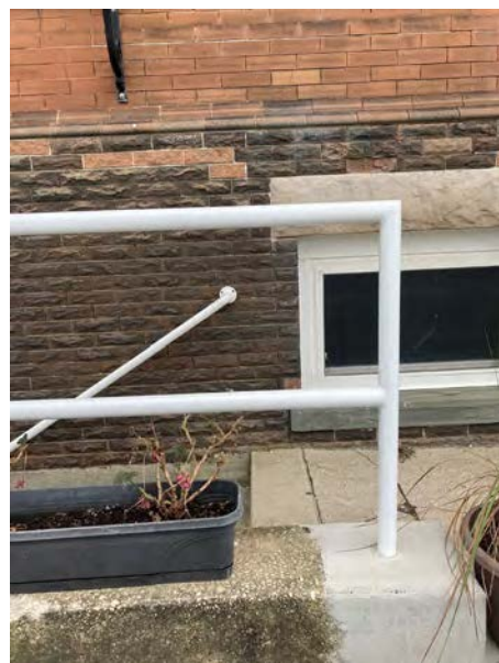
6. Rail to Below (Northeast)
