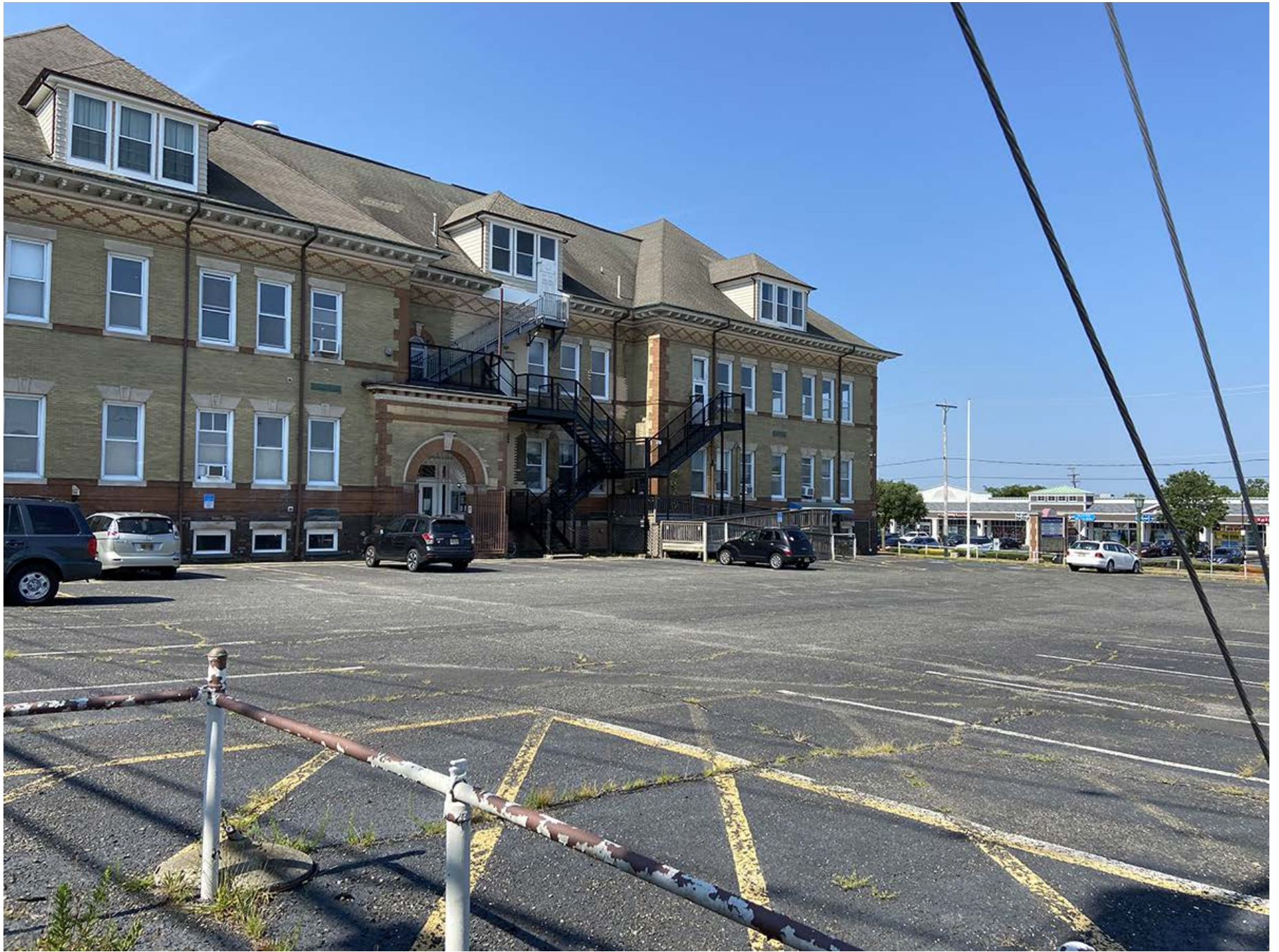
Corner View from parking area
