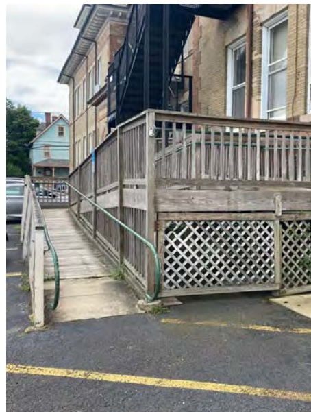
Bottom of Ramp Landing at Lot
