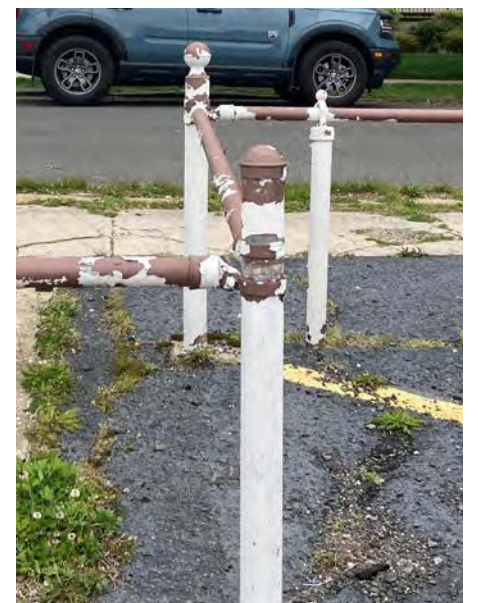
1. Parking Lot Perimeter Pipe Rail
