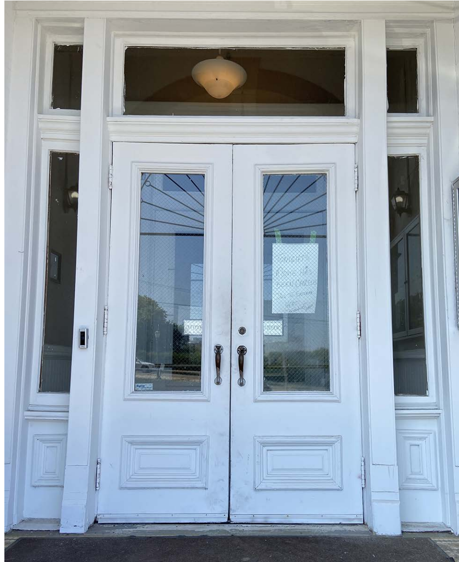
exterior of North Entryway Doors
