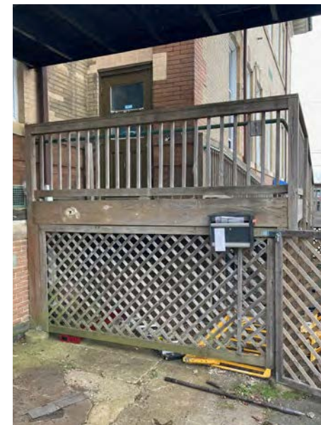
Ramp Skirt and Upper Guardrail
