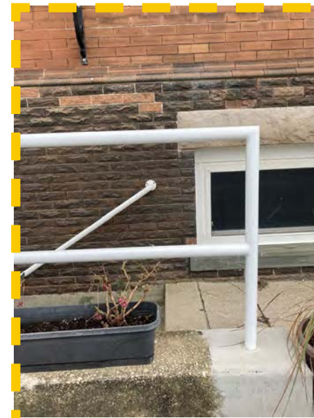
6. Rail to Below (Northeast)
