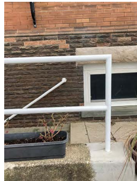
6. Rail to Below (Northeast)
