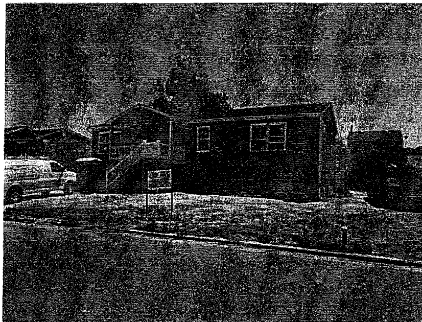
Front and East Side View of House (Looking Southerly)
